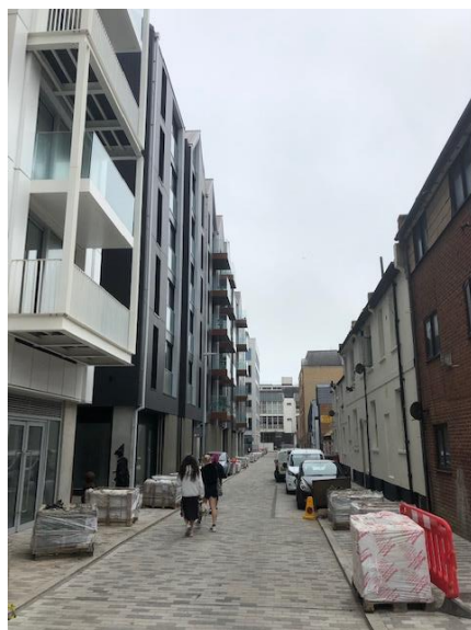
Western edge of development and public realm works, Circus Street
